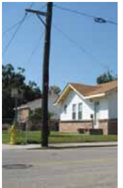
FIGURE 65. Existing conditions on Division Street. Top left and right, a lack of trees and broken, narrow, and discontinuous sidewalks create a difficult environment for pedestrians and the disabled, who are often forced to ride in the road rather than on the sidewalks. Bottom, many utility poles are located in the middle of the sidewalk, making it impossible for disabled residents to use them.
