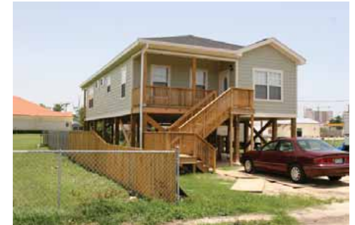
FIGURE 48. Elevated infill houses.
