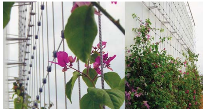
(Fig. 9) Planting screens provide shade, beauty, and security for structures and can either be attached to the structure or stand independently. (photo: Jakob®)
