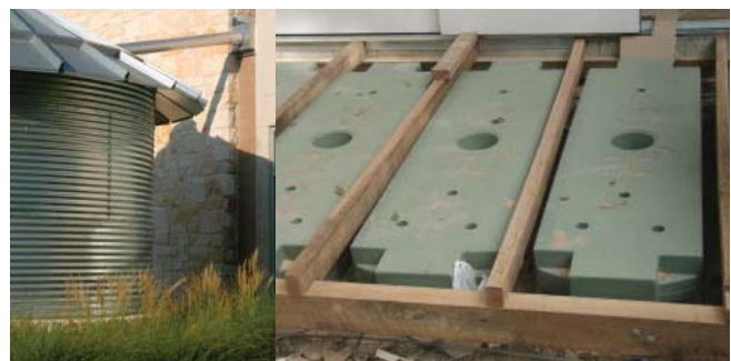
(Fig. 8) Rainwater collection systems are used to store rainwater for irrigation, and for reuse with building greywater systems.
