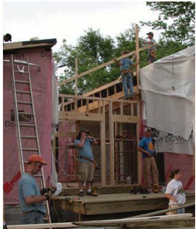
(Fig.20) Auburn University's Design Habitat students work on a project that is an example of how on-site construction can combine pieces of factory assembled modular homes to create a hybrid home.
