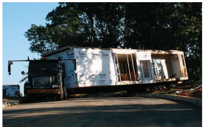
(Fig.2) The size of the unit is determined by the size of truck allowed on local roads. Site access constraints should be carefully considered before a modular home is purchased.
