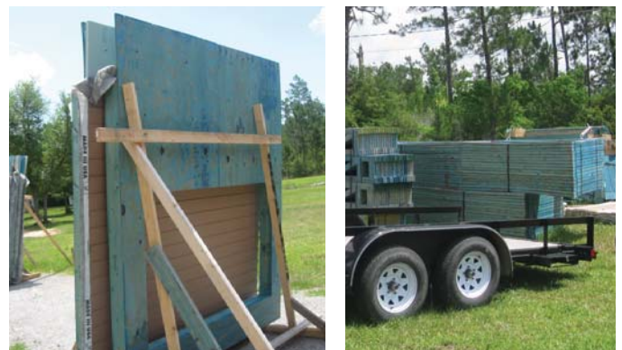
(FIG.C) KIT HOMES are delivered on-site with various parts to assemble. Included in the kit should be all the pieces needed to assemble the home.
