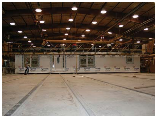
(Fig.5) Modular homes made in factories are made quickly with the help of specialized rigging and equipment.
