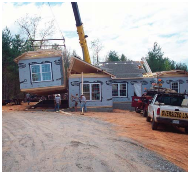
(Fig.3) The weight of modular units requires that they be lifted into place with a crane. Professional crane operators and modular installers must be used to ensure safety.
