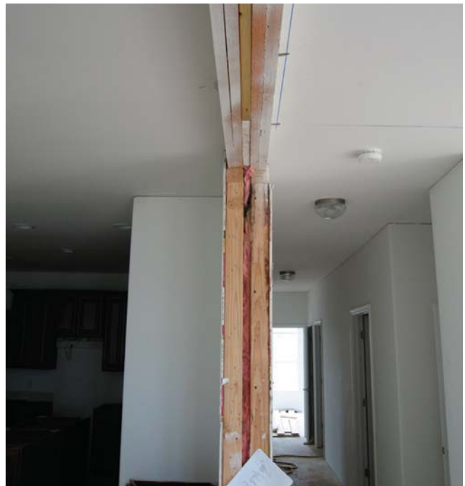
(Fig.1) Where two modules come together a "seam" wall is formed. It will need some finish work, and is often designed so that its thickness is used as an architectural element dividing two spaces such as a living and dining room.
