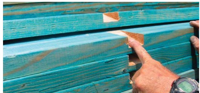
(Fig.15) Precut pieces make construction faster, but require greater precision.
