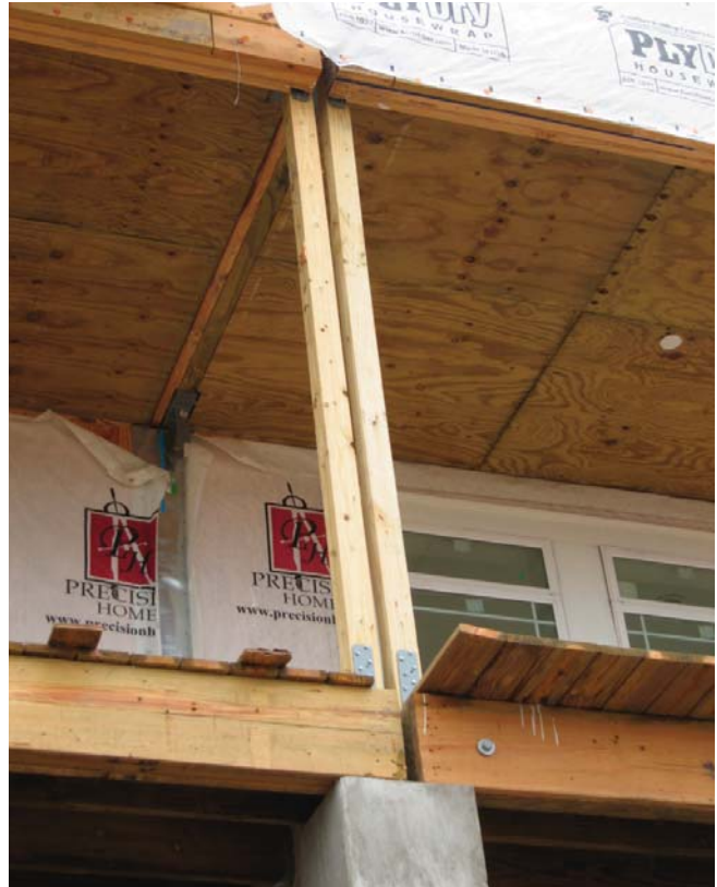
(Fig.4) Two units bears on a concrete pier. They are bolted together and fastened to the foundation.
