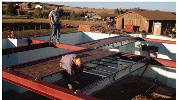
(FIG.C) SUSPENDED CAST-IN-PLACE DECKS can be used in combination with ICF walls and a concrete foundation system.
