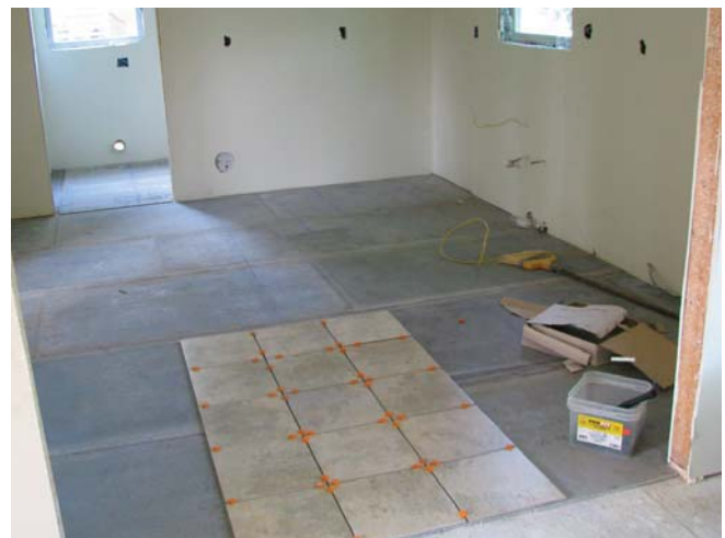
(Fig.20) Tile can be installed by professionals or homeowners. Shown here, 12" ceramic tile is being installed by skilled and unskilled volunteers.
