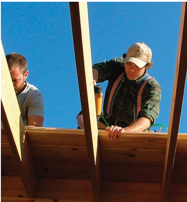
(Fig.2-3) Workers can nail through the tongue or groove into joists at an angle, which results in a single smooth surface both above and below. Two-story houses are particularly well-suited to this system.
