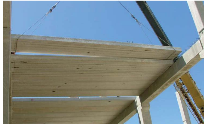
(FIG.D) PRE-CAST FLOOR PANELS can be tensioned off-site and are often hollow. Pre-cast panels can be utilized for quickly assembled, strong and fire-resistant floor systems.
