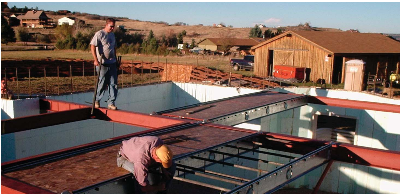
(Fig.4) Reusable steel lockbars being set into the joists. These lockbars support the plywood while the concrete is being poured and are removed after installation.
