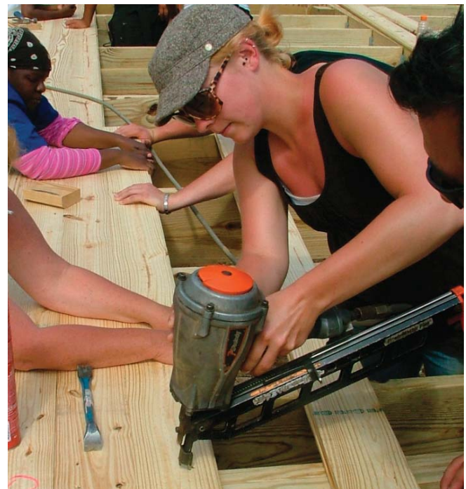
(Fig.2-3) Workers can nail through the tongue or groove into joists at an angle, which results in a single smooth surface both above and below. Two-story houses are particularly well-suited to this system.
