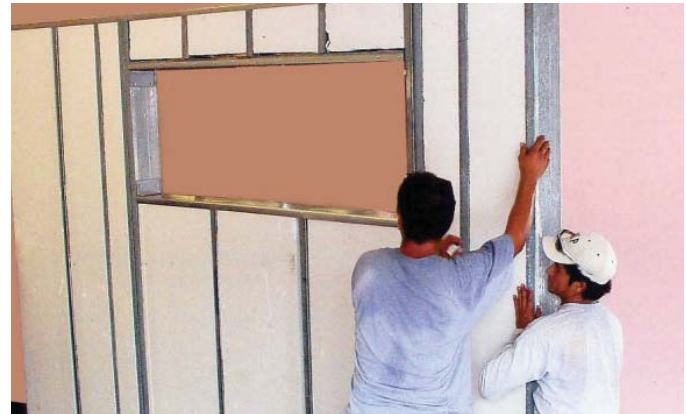
(FIG.D) FRAMED PANELS use techniques similar to standard wood or light-gauge steel framing but are built in a factory. Shown here is a steel-framed panel manufactured by Dynabilt.
