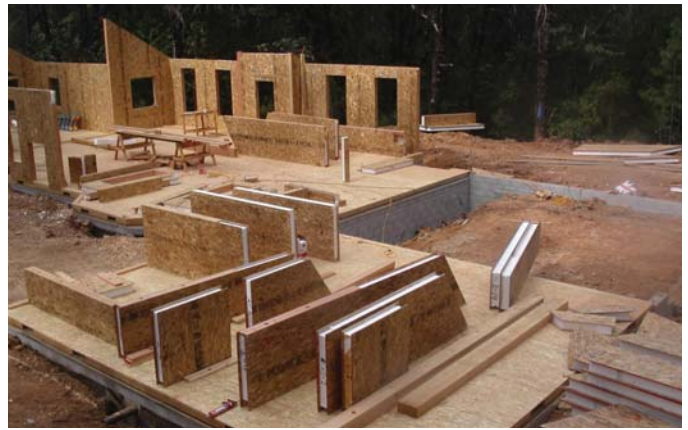
(FIG.A) PANELIZED SYSTEMS are delivered to the site as a package. Builders familiar with SIP construction can erect the structure quickly, reducing labor costs.
