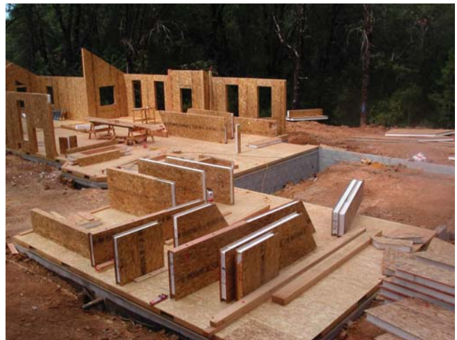
(Fig.2) Panels laid out on a building site prior to erecting the walls. A partially assembled house is visible in the background.
