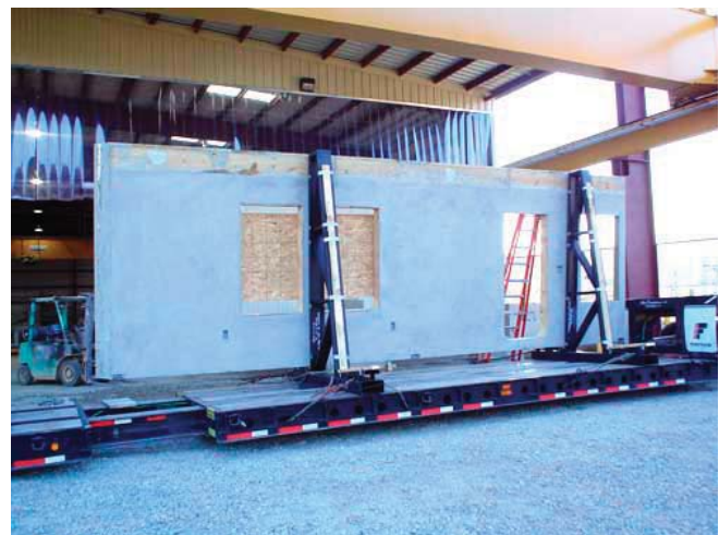
(Fig.26) Precast concrete panels loaded on a trailer for delivery.
