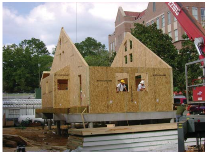
(Fig.3) A crane may be needed to lift large panels into place.
