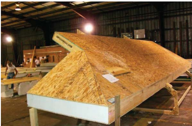
(Fig.6) Assembly of factory-made roof panels. FSU Zero Emissions House.
