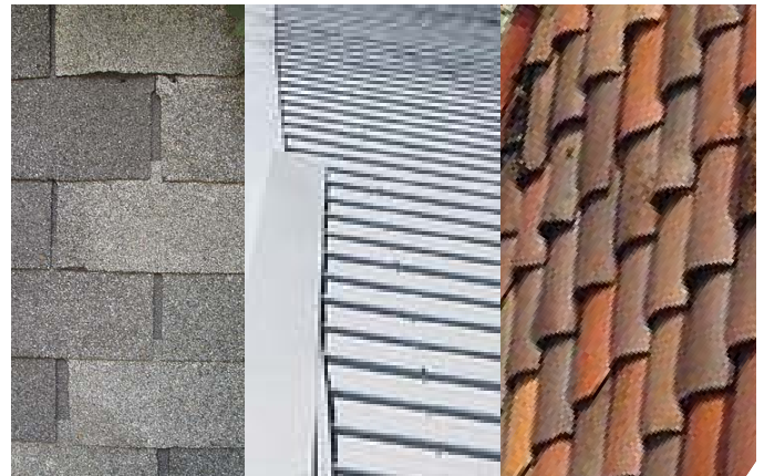
(FIG.B) Shingles, Sheet Metal, & Tile come in a variety of styles. Pictured here are asphalt shingles, metal, and clay tiles.
