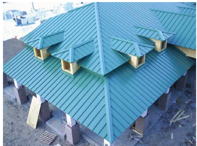
(Fig.15) Standing seam metal roofs are less common and more expensive, but have a longer life span.
