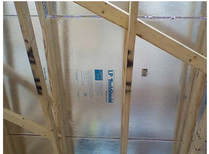
(FIG.A) Radiant Barriers are available for the underside of roof sheathing. Adding this inexpensive layer can reduce Mississippi cooling bills by 15%.
