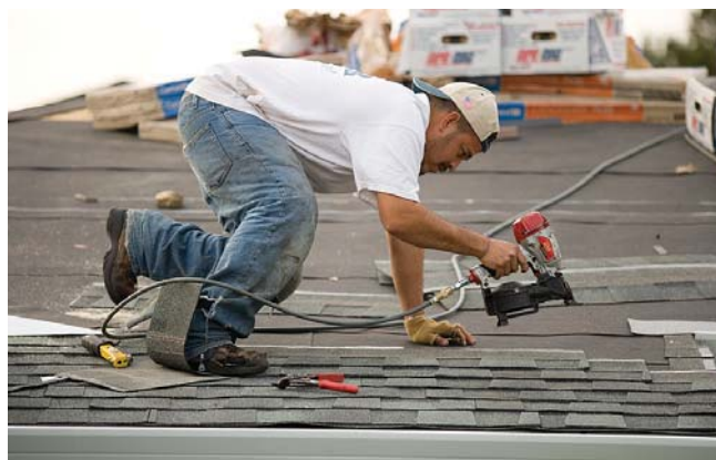
(Fig. 8) A roofing installer nails down strips of asphalt shingles.
