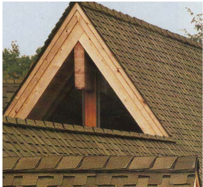
(Fig.9) Architectural-style asphalt shingles are a more expensive, but more textured, alternative to a flat shingle.
