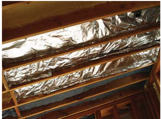
(Fig.6) Radiant barriers are often installed between roof rafters. This is an example of a radiant barrier type that could be installed in an existing building.
