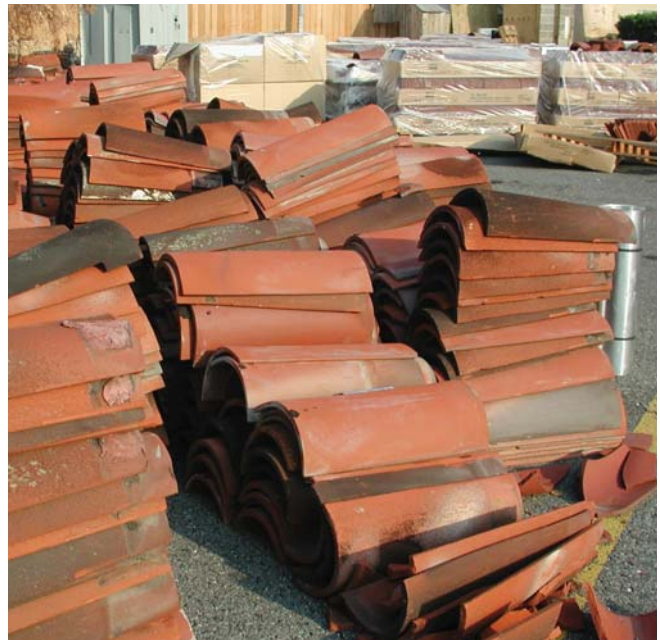
(Fig.16) Tile will be delivered to the site on pallets. The weight of tile makes them difficult to move around on site.
