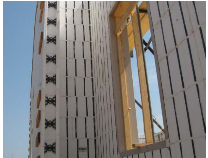
(FIG.A) INSULATED CONCRETE FORMS (ICF) is often manufactured with plastic vertical strips for adhering exterior finish material.
