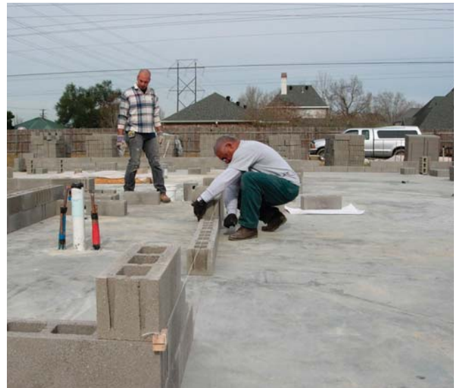
(Fig. 8) A stringline is used to lay the first course of a CMU wall.
