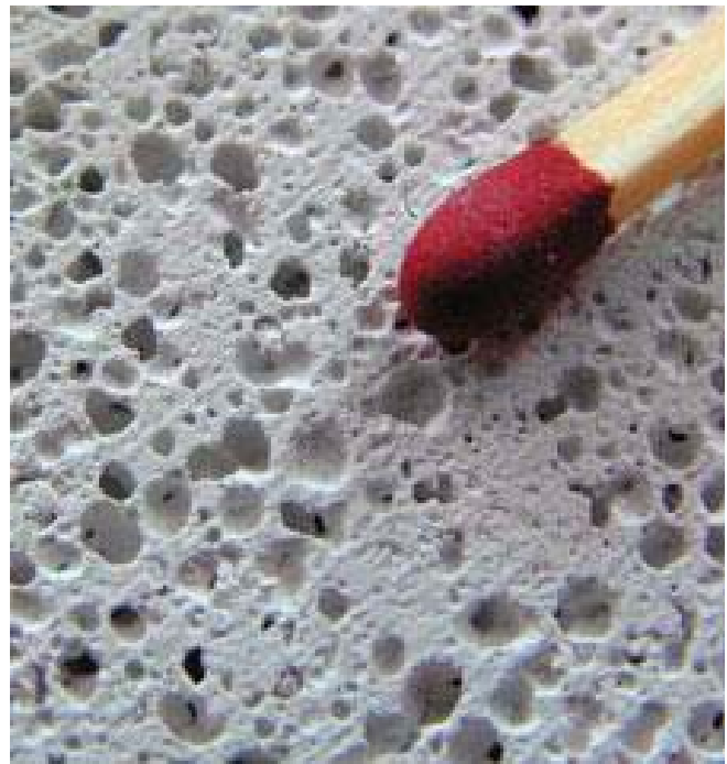
(Fig. 15) Tiny hydrogen bubbles are created when the concrete is combined with aluminum powder.
