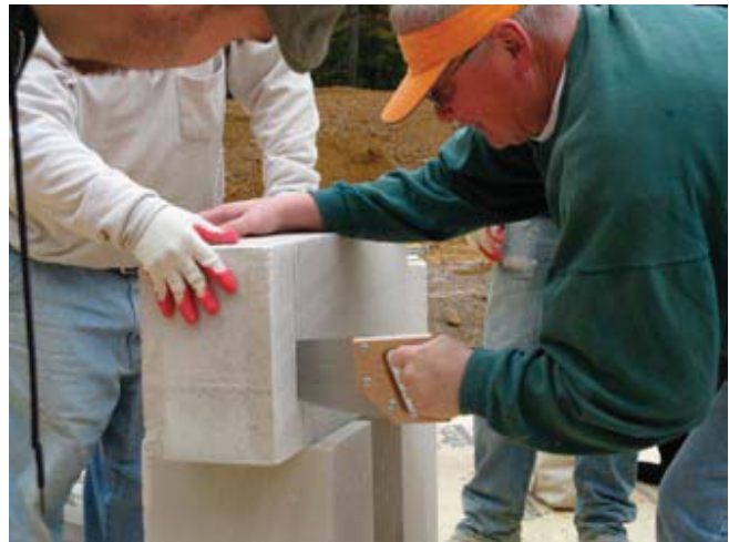
(Fig. 17) AAC blocks are easily cut on-site without the need for special saws or blades.
