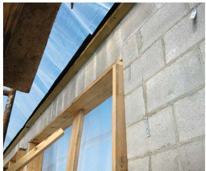
(Fig. 10) Reinforced lintels are used to span window and door openings in walls. Above, the CMU blocks are turned vertically so rebar can be set horizontally through the cavities.
