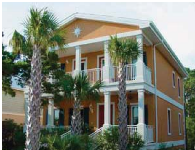
(Fig. 5) ICF walls offer superior acoustic insulation, making them a good choice for partition walls in multi-family projects.
