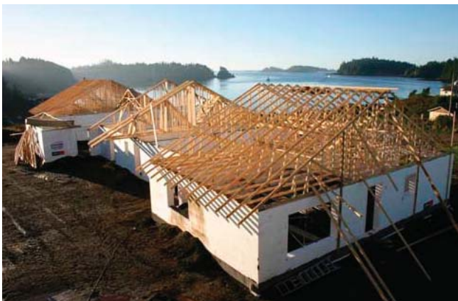
(Fig. 1) Insulated Concrete Formwork is most commonly used in wall construction and combined with other systems, such as wood stick-framing for the roof structure, as shown above.
