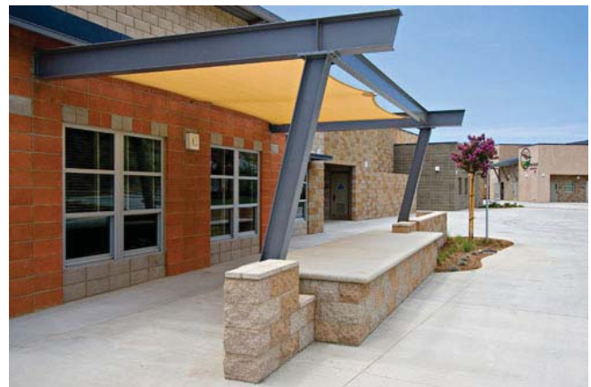
(Fig. 9) CMU wall construction is commonly found in institutional applications, such as this school shown above.
