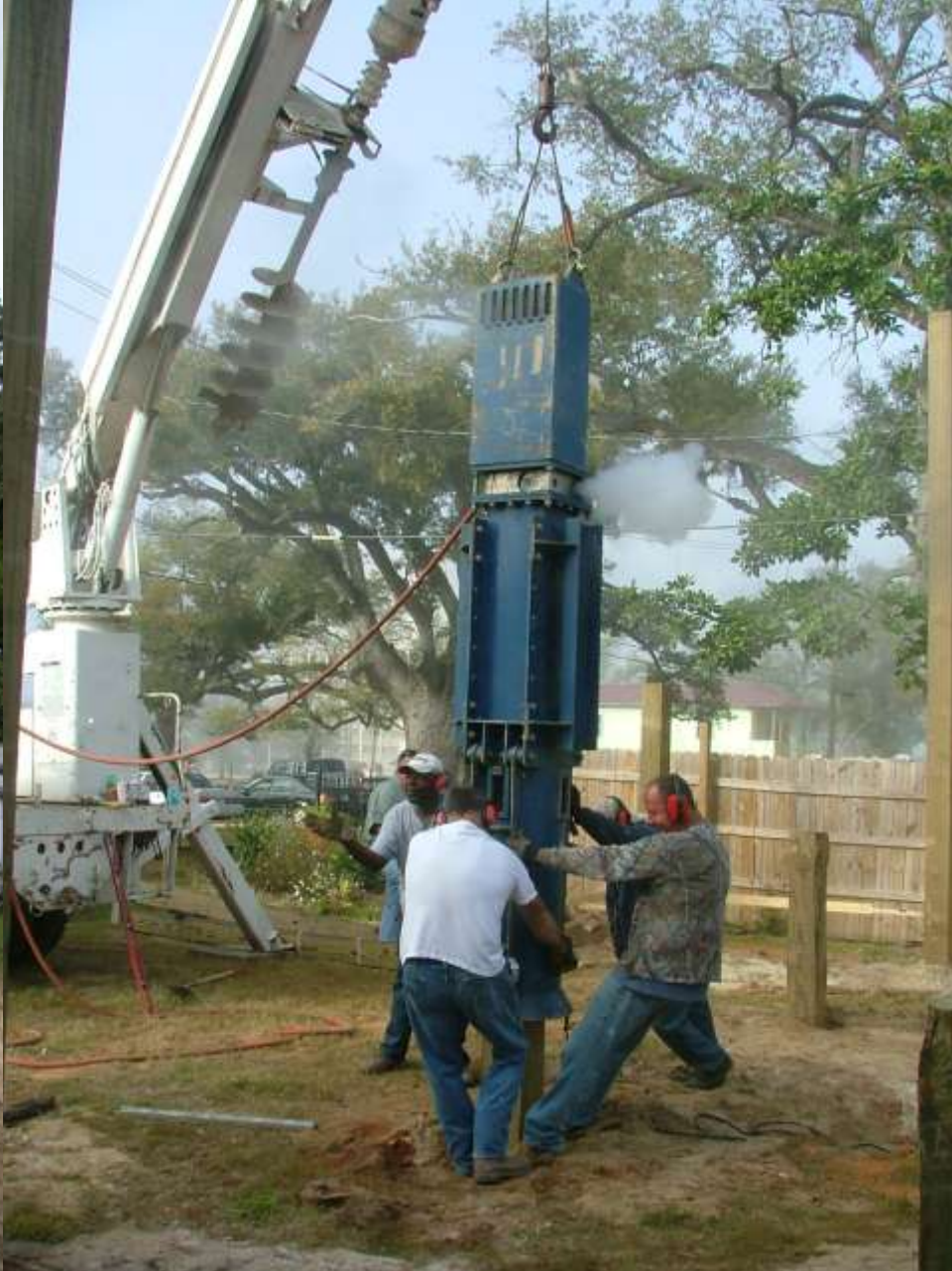
DEEP FOUNDATIONS- DRIVEN WOODEN PILES
